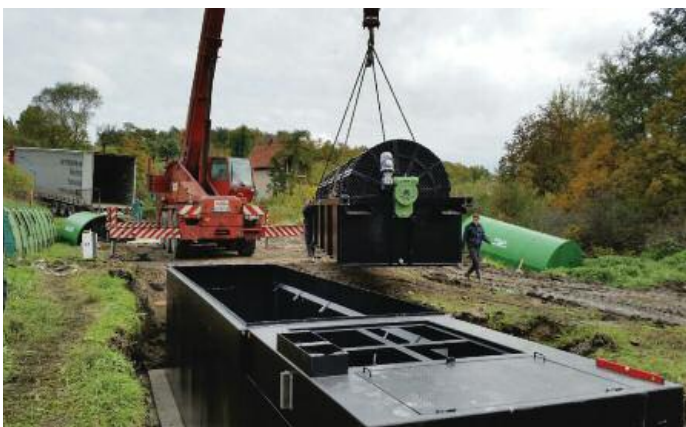
Ugradnja biorotora u raznim uvjetima za vaše domove, stambena naselja, turistička naselja i gospodarske objekte Installation of biorotors in various conditions for your homes, residences, tourist resorts and commercial housing
