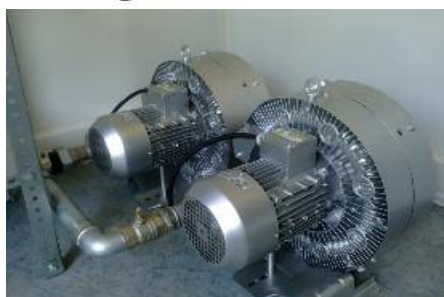
PUHALA U RADU / BLOWERS IN OPERATION
