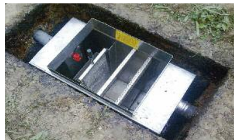
Prikaz ugradnje mastolova Installation of a grease trap
