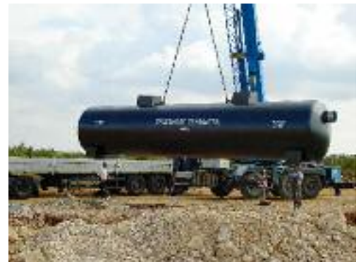
Assembly of special separator type TEHNIX
