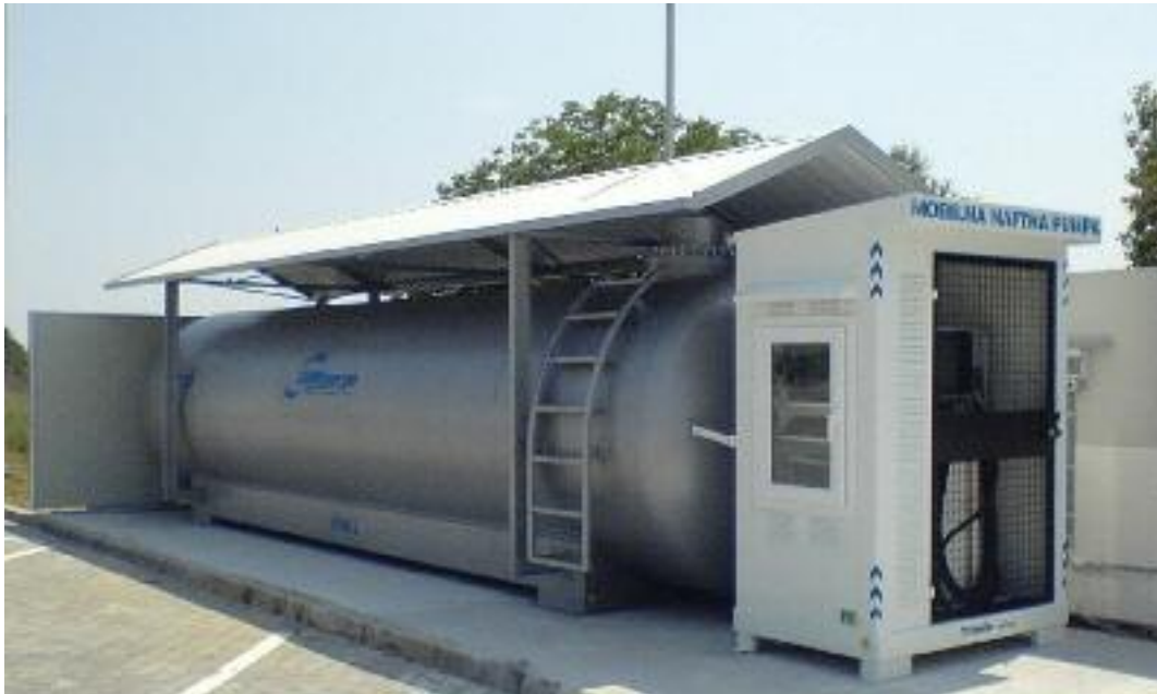
MNP with computer equipment with the volume of 25,000 liters
