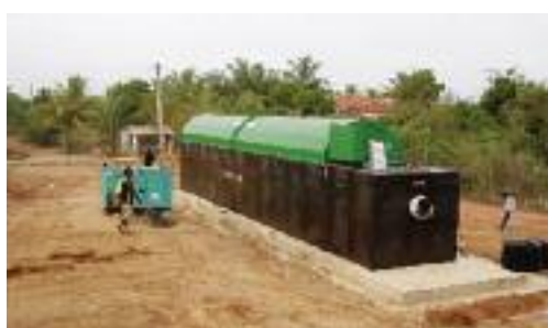
Montage of BRT-1500 in Sri Lanka
