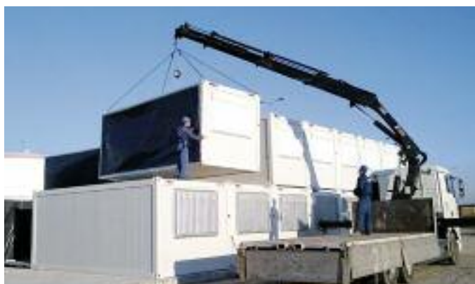
Assembly container settlement on site
