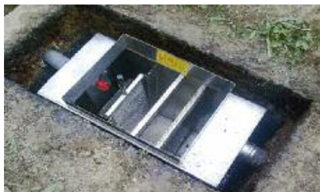
Installation of the grease-trap
