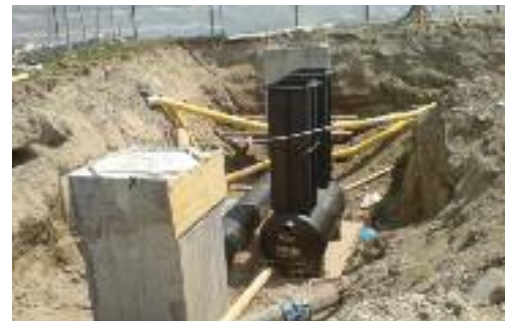
Installation of the special separator
