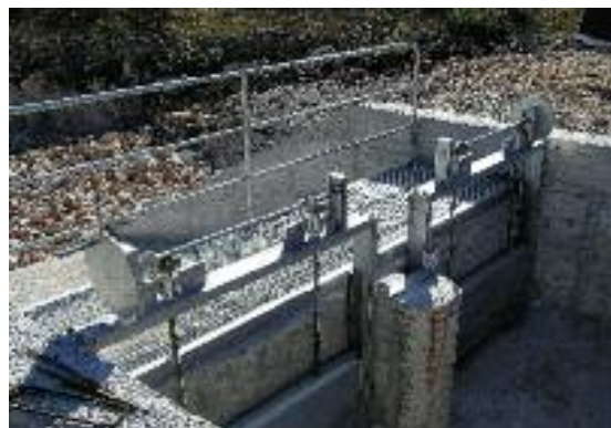
Overview of installed stoppers on-site
