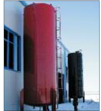
Vertical cisterns according to DIN 6618
